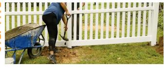
Cover the rest of the footing with dirt. Add caps to the top of the fence posts and the fence is complete!
